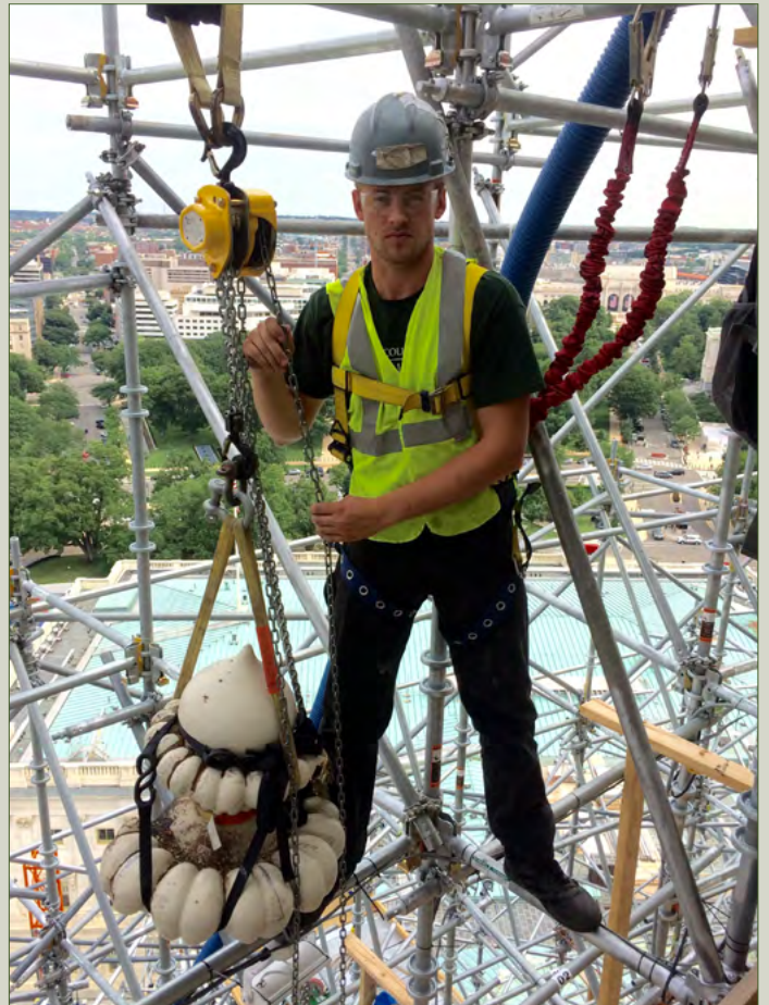
REPAIRING THE U.S. CAPITOL DOME IN WASHINGTON, DC
